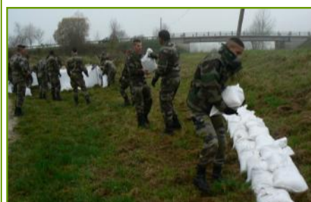
Dike strengthening in Lacroix-sur-Meuse.
