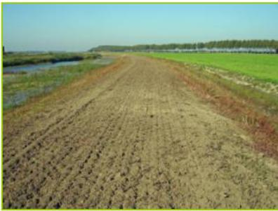
Here we're standing on the new summerdike; on the left a new bypass was dug out; the old summerdike is situated behind the reeds far left. The poplars on the right mark the limit of the former valley of the Steenbergse Vliet. Just right of the new summerdike is a drainage ditch to the profit of the farmer, who can still grow corn on the arable fields.
