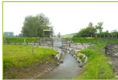
*Infrastructure to control discharges including a gate and a low-water bed*
