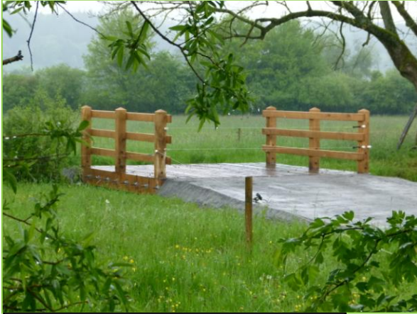
Pontoon built in order to avoid damage of the banks by cattle tramping
